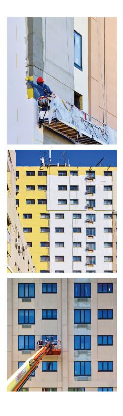
The windows were also replaced, which proved to be an interesting challenge. According to applicator Dinko Beharic of Rima Designs, LLC, when the carpenters were removing the windows, his team would follow in and apply a double coat of Sto Gold Coat, the ready-mixed fluid applied air and moisture barrier membrane, sealing the windows to eliminate any potential leaking. Doubling the Sto Gold Coat also made it impossible to see the brick through it.
