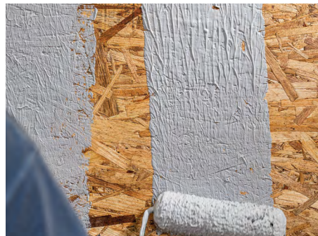
Oriented strandboard (OSB) and plywood share properties of both CMU and ASTM C1177 sheathing. Neither as smooth as gypsum sheathing nor as porous and moisture absorbent as CMU, on wood-based substrates thinner membranes provide fast drying. Weathered wood-based sheathing may require touch-up or a second application of Sto AirSeal to obtain a void and pinhole-free membrane.
