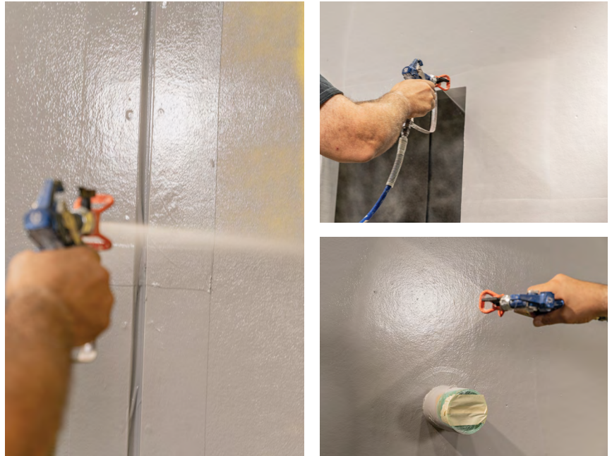
StoGuard Detail Components receive a fully compatible overcoat of Sto AirSeal for extra protection where it is needed most.
