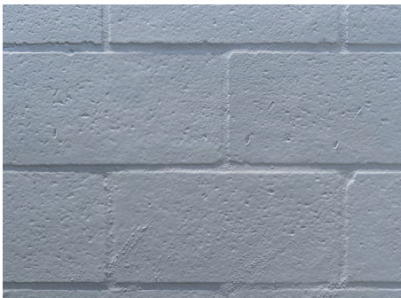
Concrete masonry units (CMU) are rough and porous, and draw moisture out of water-based products, helping them dry quickly. High-build membranes are well suited to the rough CMU surface.
