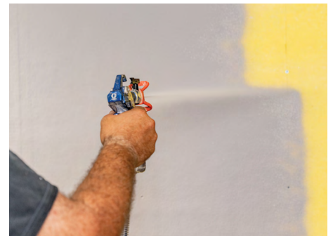
ASTM C1177 gypsum sheathing is smooth and nonporous with limited moisture absorption. High membrane thickness can extend drying time. Already an air barrier material and much less prone to pinhole formation, gypsum sheathing can be effectively protected with a thinner, single coat Sto AirSeal membrane.
