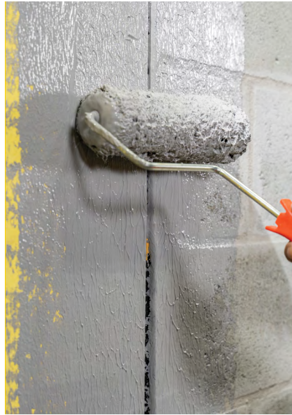
StoGuard Detail Components receive a fully compatible overcoat of Sto AirSeal for extra protection where it is needed most.
